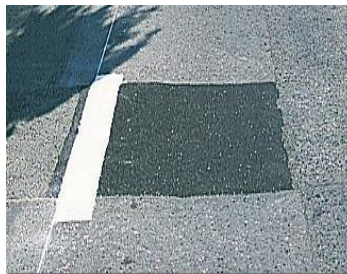
Restoration after Utilities works
